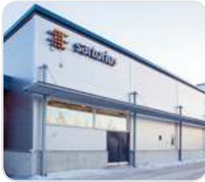
The factory in Kajaani, Finland.
